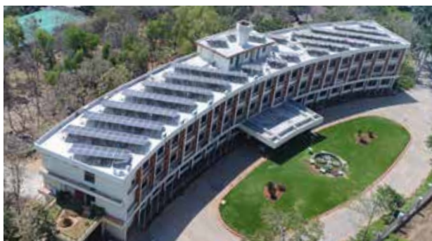
200 KW Solar Plant on the roof top of admin building at Mysuru Complex
