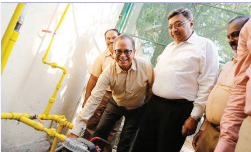
Inauguration of Bio-gas Plant at Bengaluru Complex in the presence of Shri Subhash Chandra, IAS, Secretary Defence Production, GoI.
